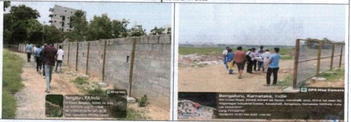
Work yet to be completed
